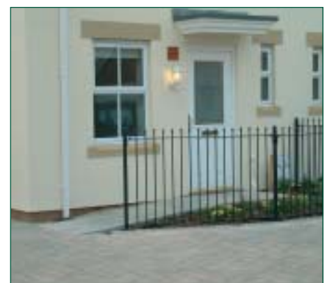
Ramp with Railed Front Garden
