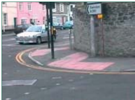
Tactile Warning Surface at Pedestrian Crossing
