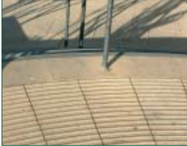
Tactile Paving above steps
