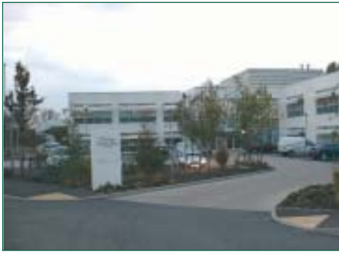
Tactile Warning Surface at Road Edge
