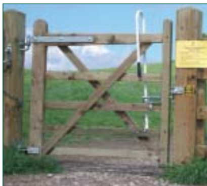
Accessible Gate (Centrewire)
